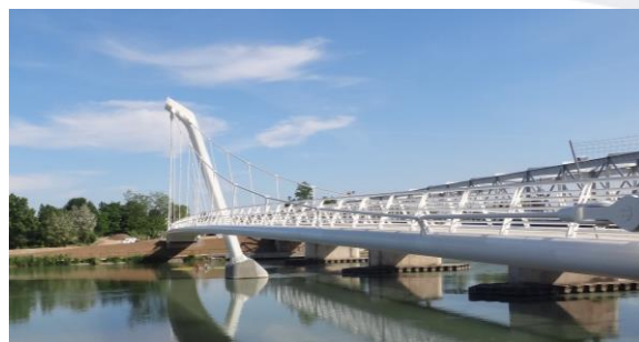
Decines Bridge, France
