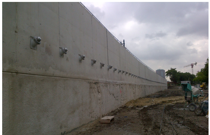
Tie-back reinforced wall
