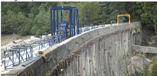
Installation with winch and guide
