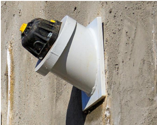
Anchor head equipped with an angular chair
