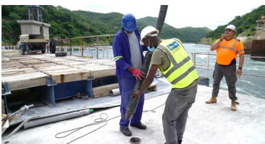
Installation by crane (with lifting point)
