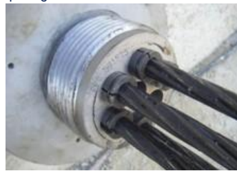
Threaded block before stressing
