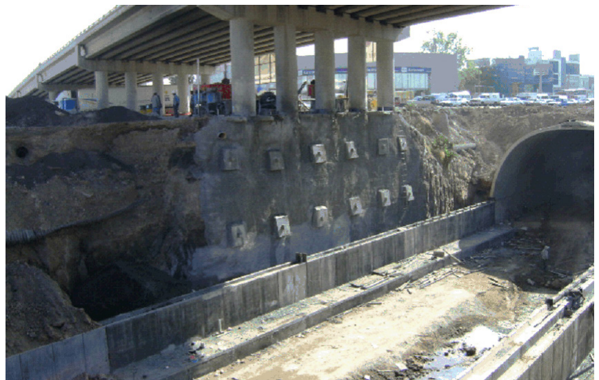
Slope stabilization under bridge foundation
