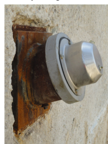
Head with temporary protection and bearing chair
