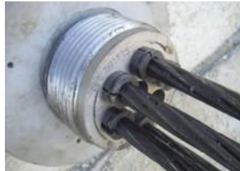
Threaded block before stressing
