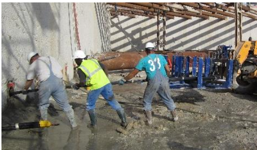
Installation with an uncoiler
