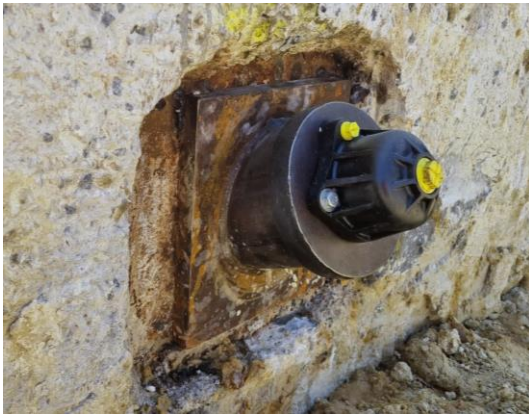
Anchor head equipped with an angular chair
