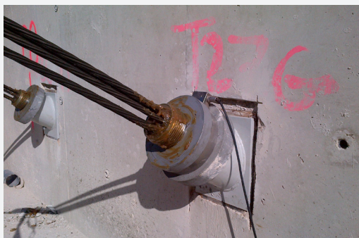
FreysCell system fitted to a Freyssinet 4C15 tie rod
