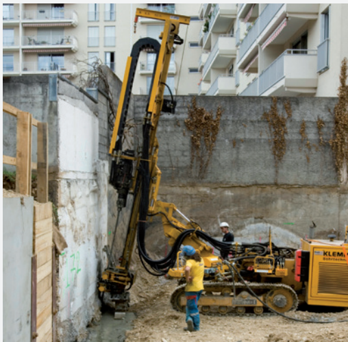
Installing a micropile
