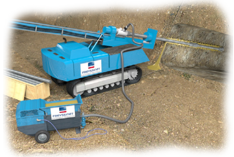
Simultaneous grouting and drilling
