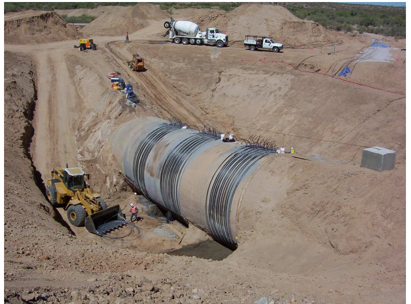
Reinforcement of a buried pipeline
