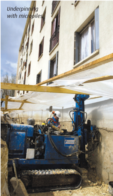
Underpinning with Fondapieu
