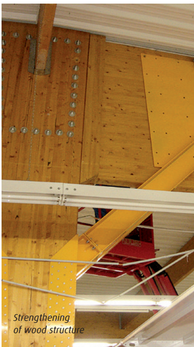
Floor strengthening with Foreva®TFC
