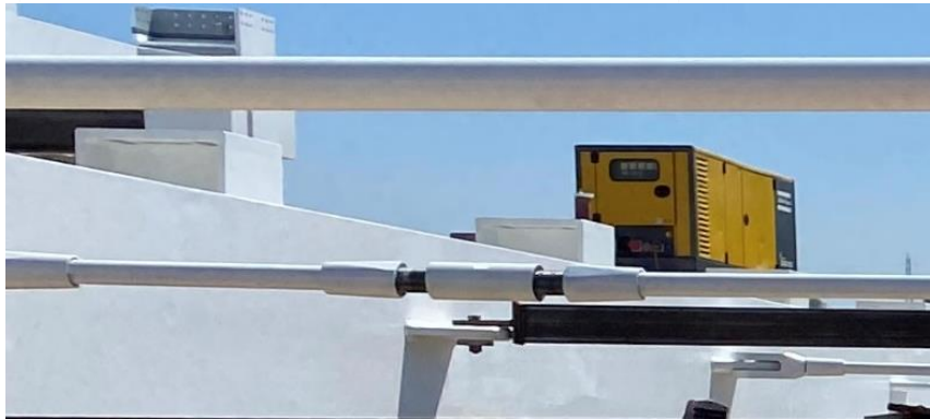
Lock nuts open for by-pass tooling installation
