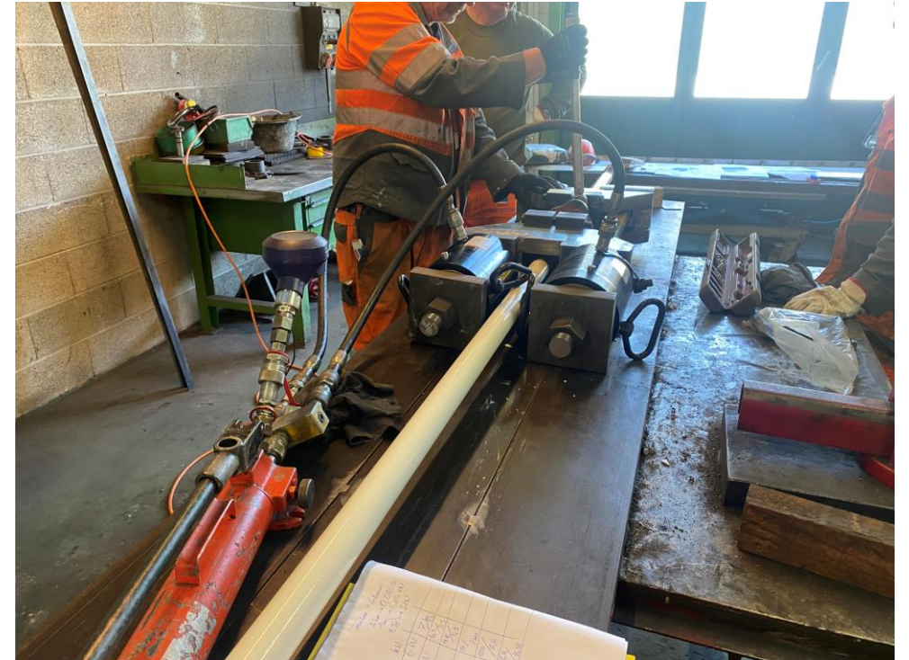
Control & adjustment tool trial installation
