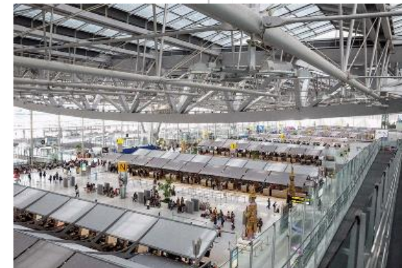
TRUSS STIFFENING ELEMENTS
