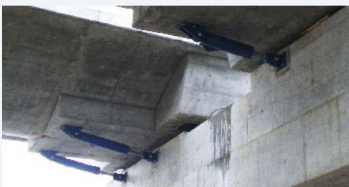
ISOSISM® FD installed underneath a bridge deck
