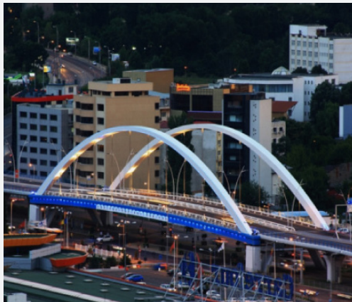
Arch Bridge - Basarab - Bucharest
