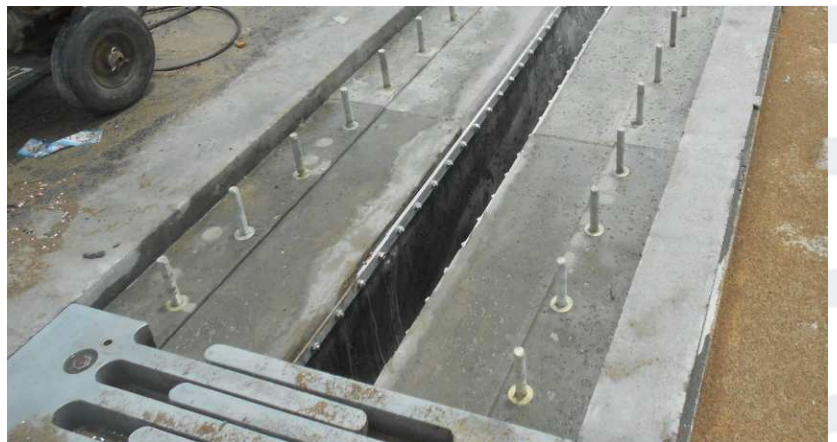
Details of the elastomeric membrane
