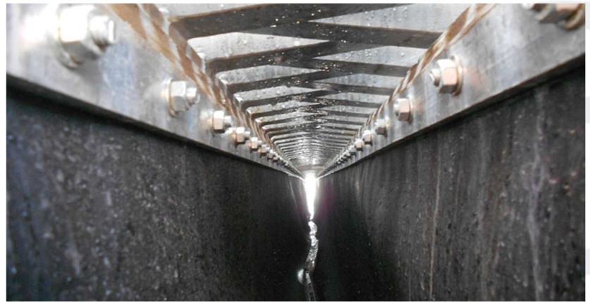
Close-up view of WP500 elastomeric membrane – Abidjan Riviera Marcory
