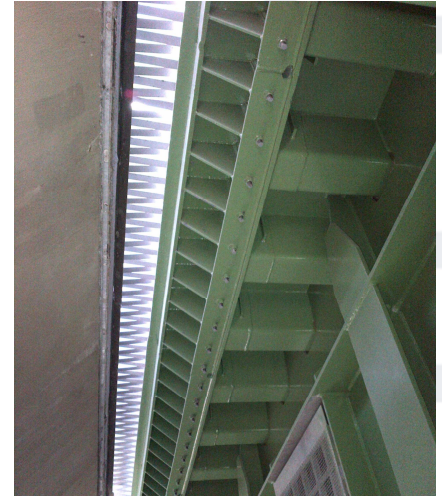
WP550 connected to an orthotropic deck, Szébbény (Hungary)
