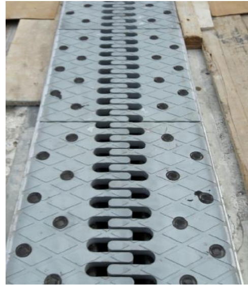
Figure 33 : Photos of a WP 180 and WP160 with 2 rows of fixings and groove
