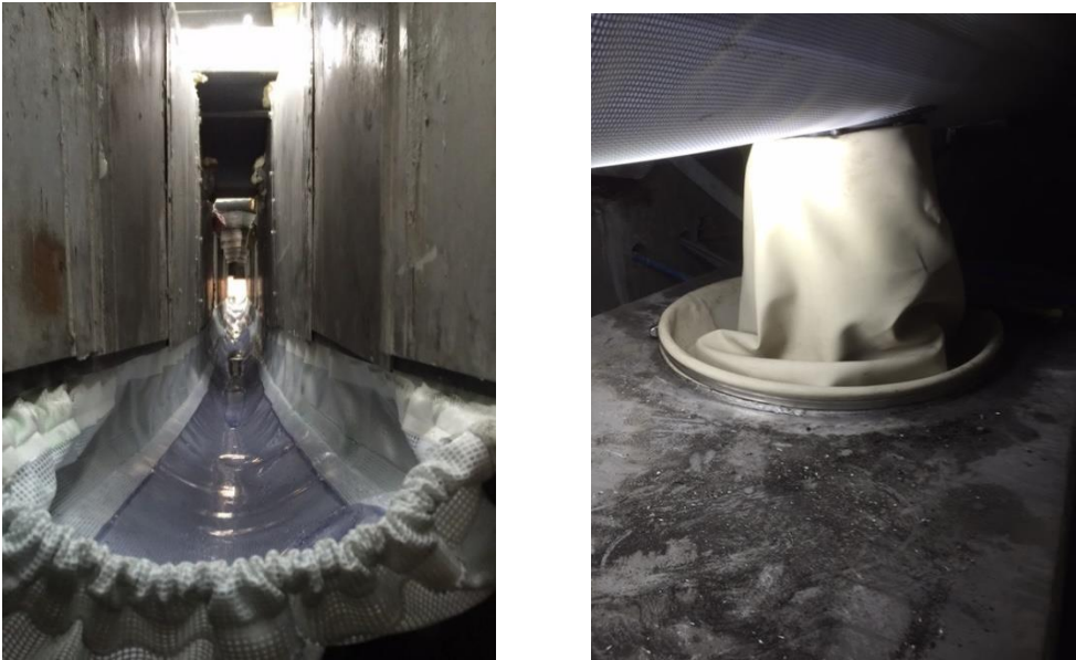
Figure 15 : Removable elastomeric membrane
