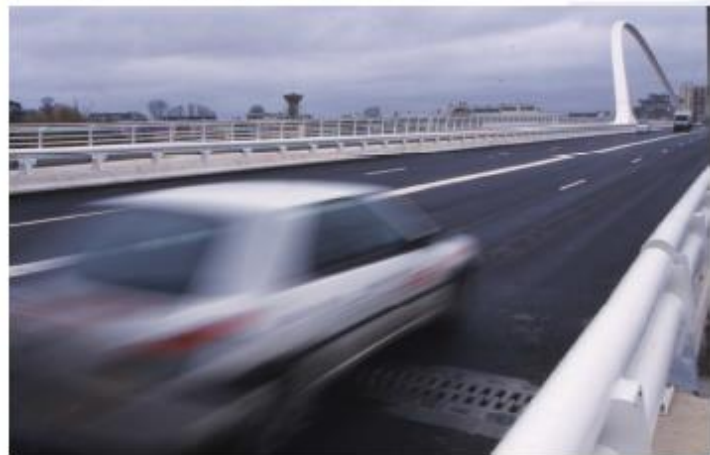
Europe bridge, Orléans (France) equipped with WP 250
