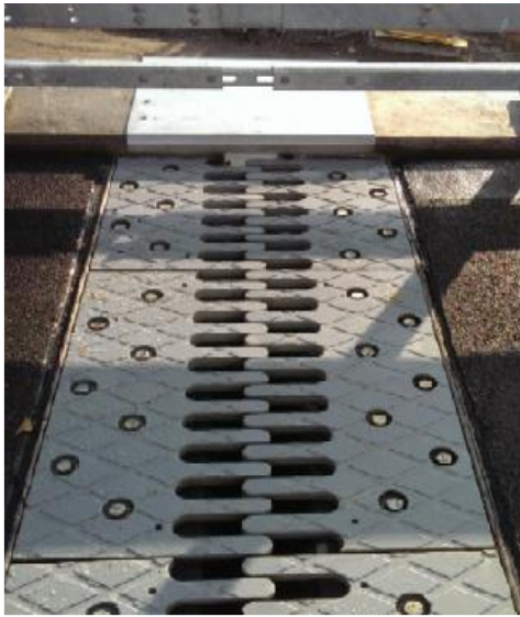
Figure 33 : Photos of a WP 180 and WP160 with 2 rows of fixings and groove
