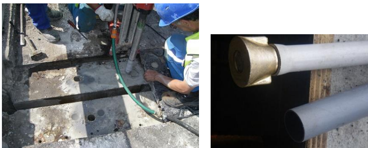
Figure 37 : Photo of a coring and cone fixing
