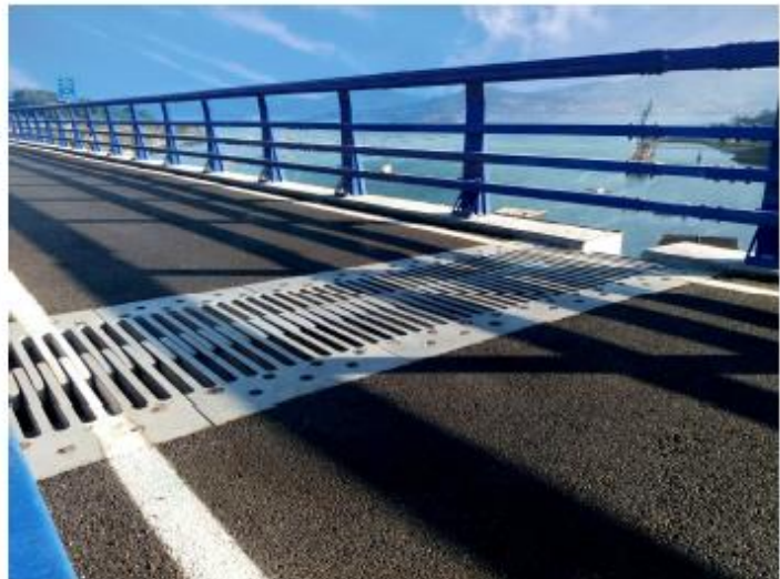
Rande Bridge (Spain)
