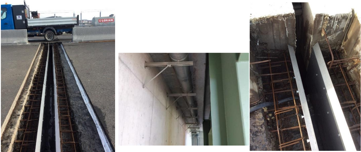
Figure 16 : Stainless steel membrane with rainwater recovery in a gutter
