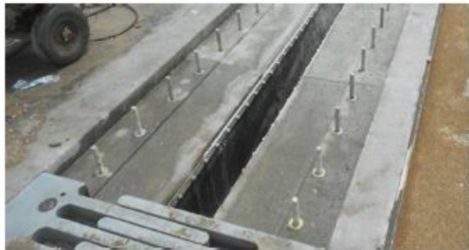
Details of the elastomeric membrane
