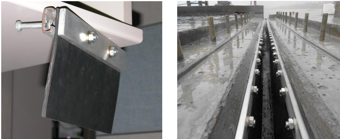
Figure 13 : Standard elastomeric profile with rail Halfen
