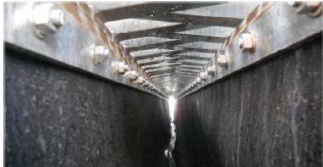
Close-up view of WP500 elastomeric membrane - Abidjan Riviera Marçay
