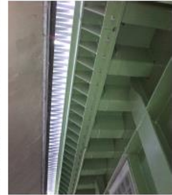
WP550 connected to an orthotropic deck, Széchenyi (Hungary)
