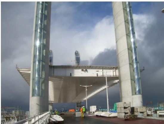
Chaban-Delmas lifting bridge (France), equipped with Wd110
