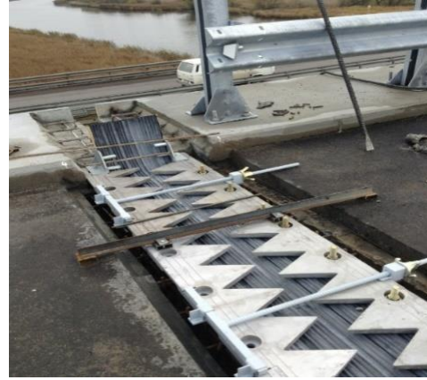
Figure 16 : Installation of the Wd joint
