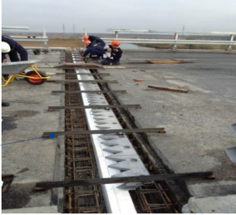
Figure 16 : Installation of the Wd joint
