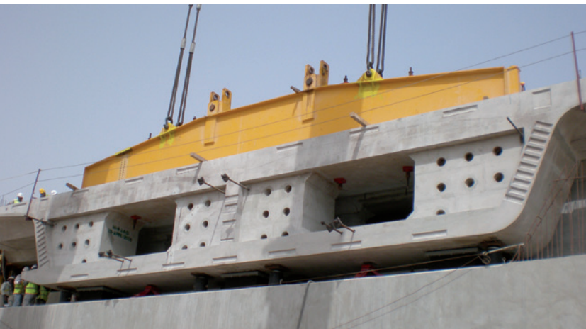
Lifting : prestressed connection between a segment and a beam.
